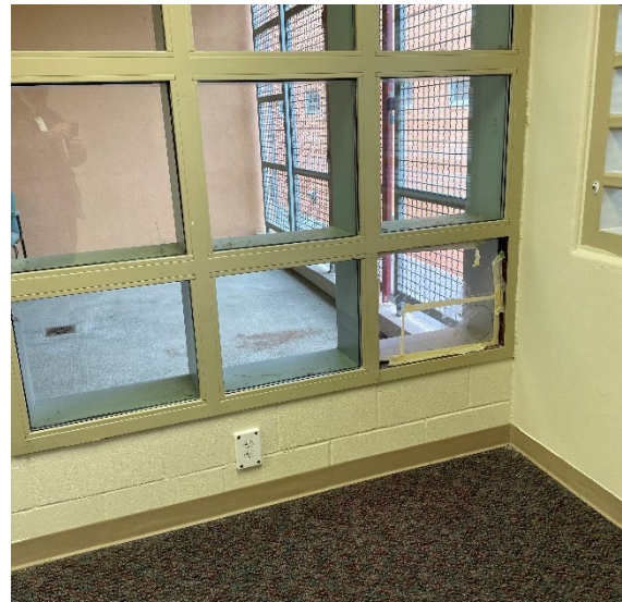
Figure 1: Window and frame deterioration at covered recreation areas.
