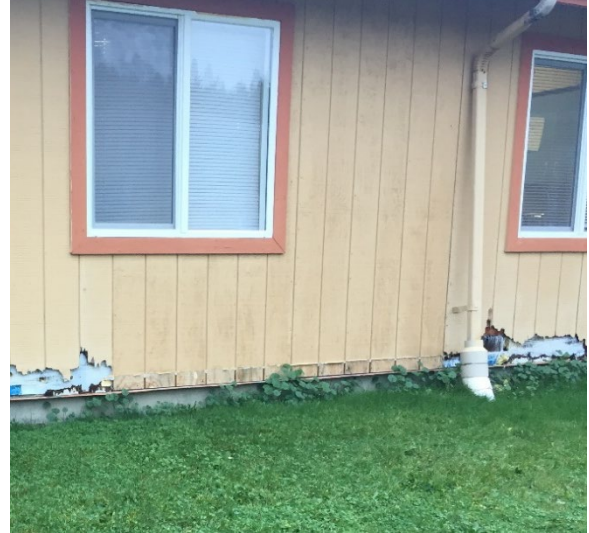
Figure 2: Deterioration of exterior cladding and insulation on Redwood Housing
