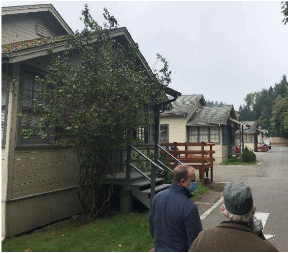
Figure 6 Image of the existing ATP building
