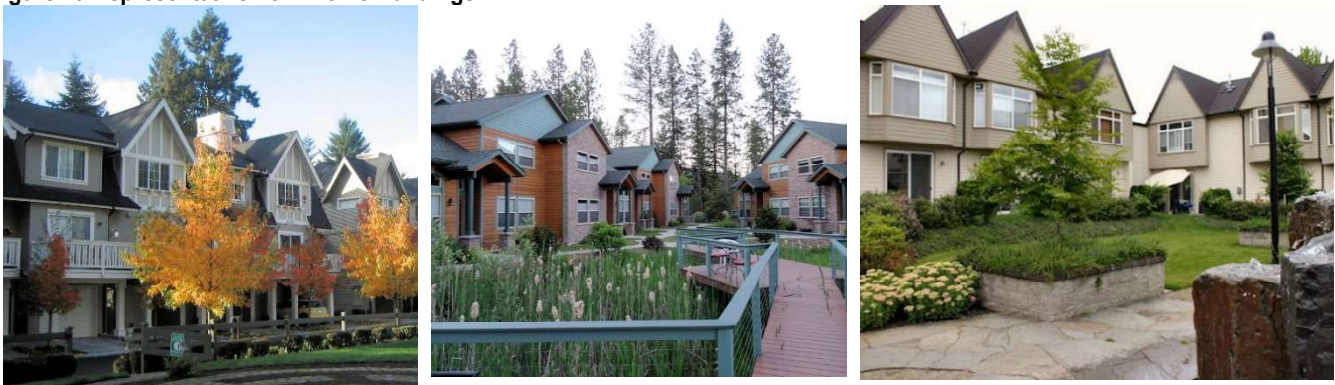
Figure 19 Representative Townhome Buildings
