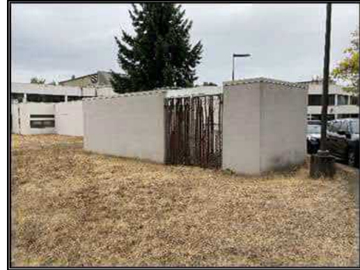
East Campus Well House
