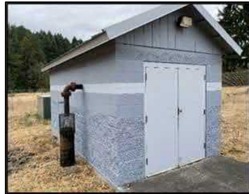
Farm Well House
