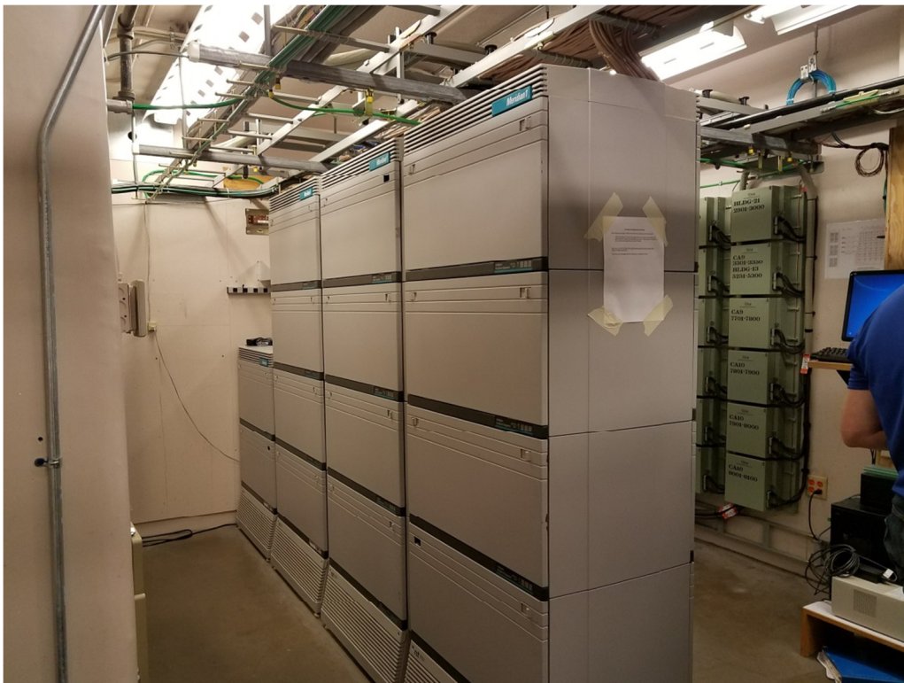
Photo 1: Existing Nortel PBX
