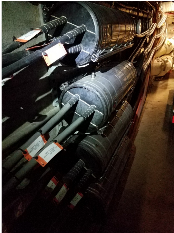
Photo 5: Steam Tunnel entrance from Building 18
