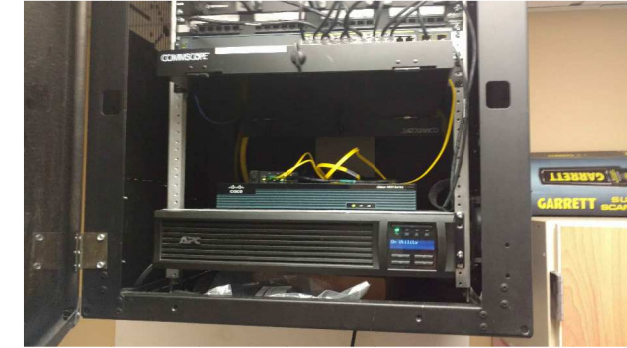
2 BUILDING 17 FIRST FLOOR IDF RACK
