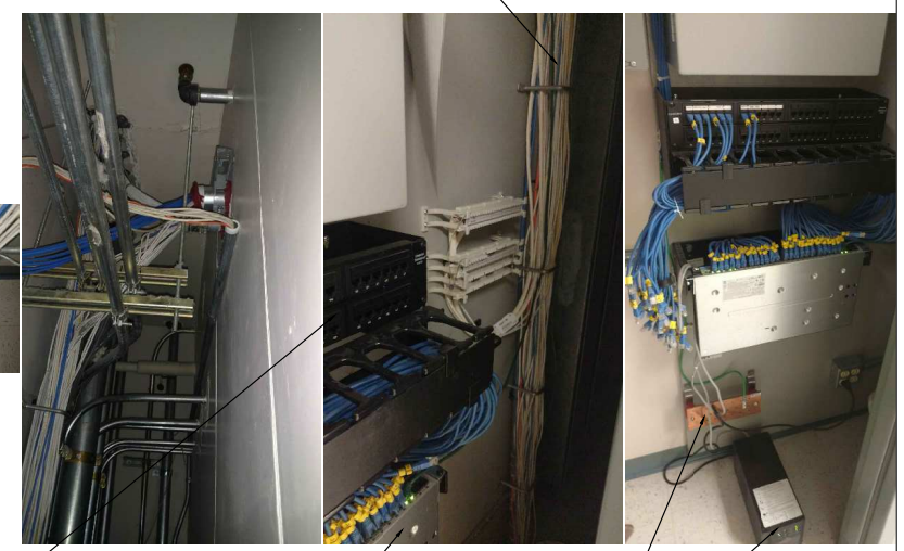
2 BUILDING 20 FIRST FLOOR IDF ROOM
