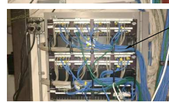
3 BUILDING 29 IDF CLOSET
