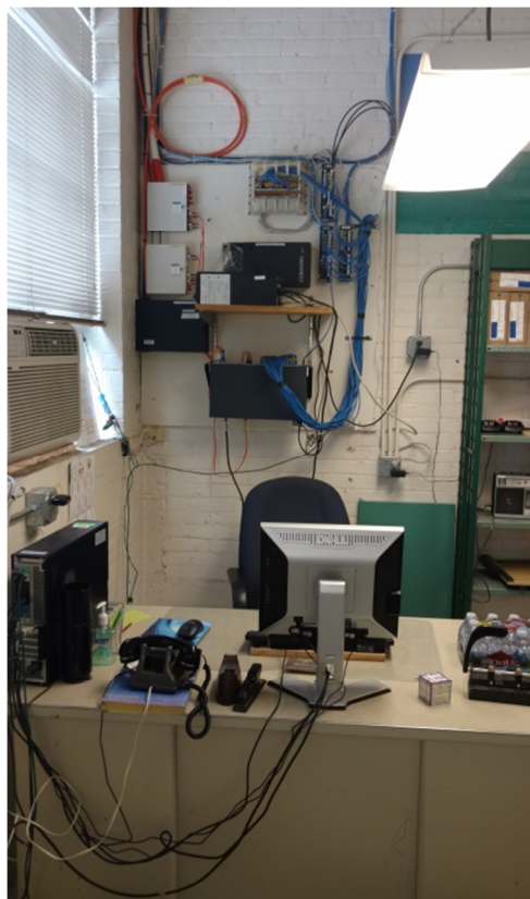
Photo 2: Example of shared Telecommunications Space - Machine Shop
