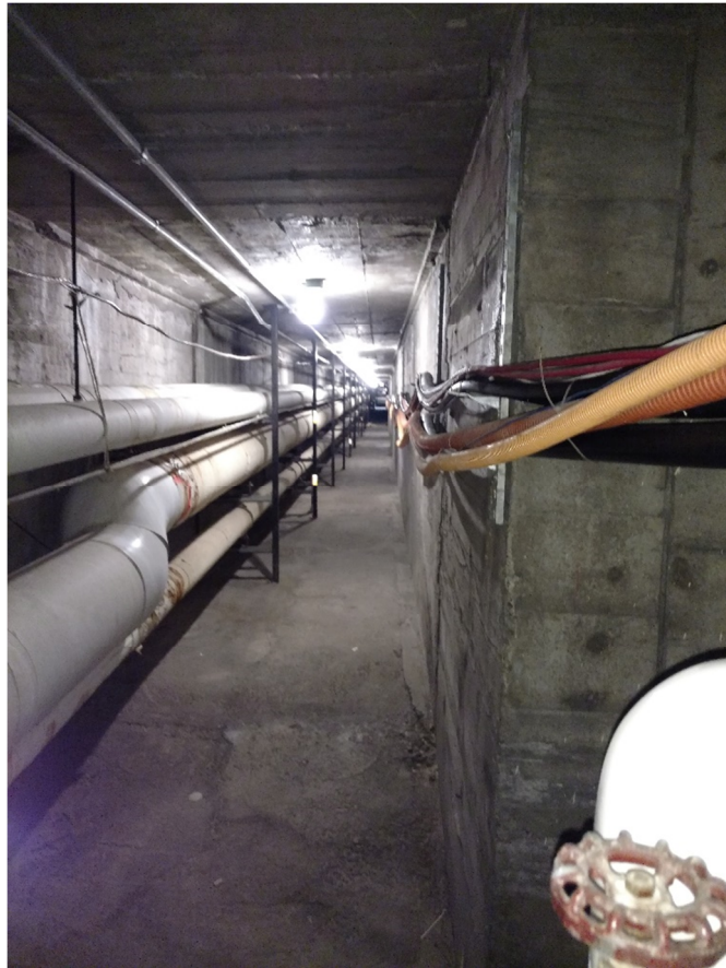
Photo 4: Tunnel from Building 9
