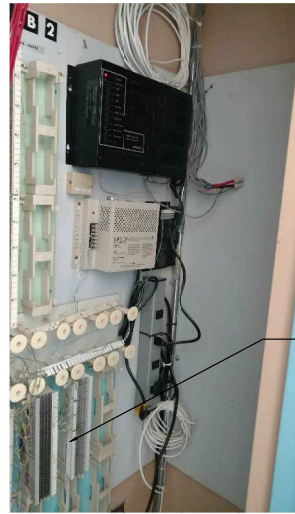
2 BUILDING 29 IDF CLOSET
