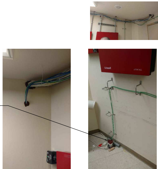
1 BUILDING 21 FIFTH FLOOR IDF ROOM
