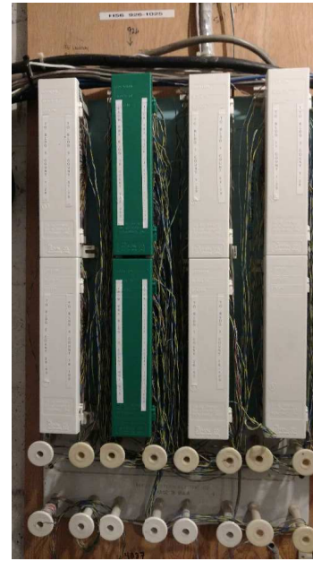
3 BUILDING 4 TELEPHONE BACKBOARD
