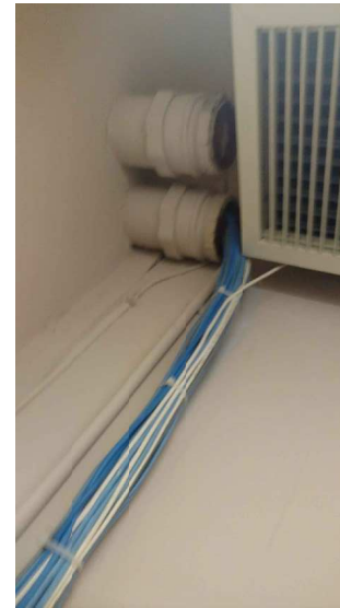
1 BUILDING 19 TELECOM IDF ROOM
