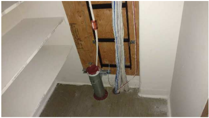
1 BUILDING 9 RM 337 TR ROOM
