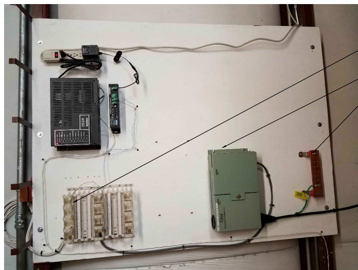
2 BUILDING 32 TELEPHONE BACKBOARD
