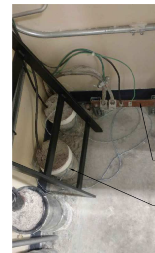
GROUND BAR ENTRY CONDUIT
