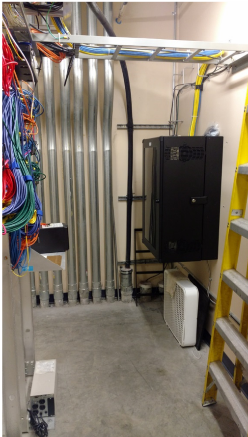
Photo 3: Building 28 Telecommunications room F102
