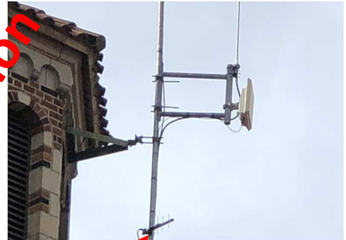
Bell Tower directional antenna to the east.
