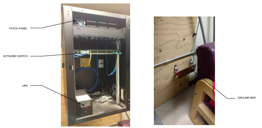
BUILDING 21 FOURTH FLOOR IDF ROOM
