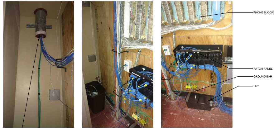
1 2 3 BUILDING 16 ELECTRICAL CLOSET 232 ELEVATION
