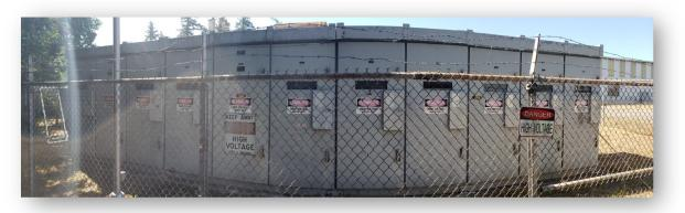
Photo 2: Main Distribution Equipment with Main-Tie-Main
