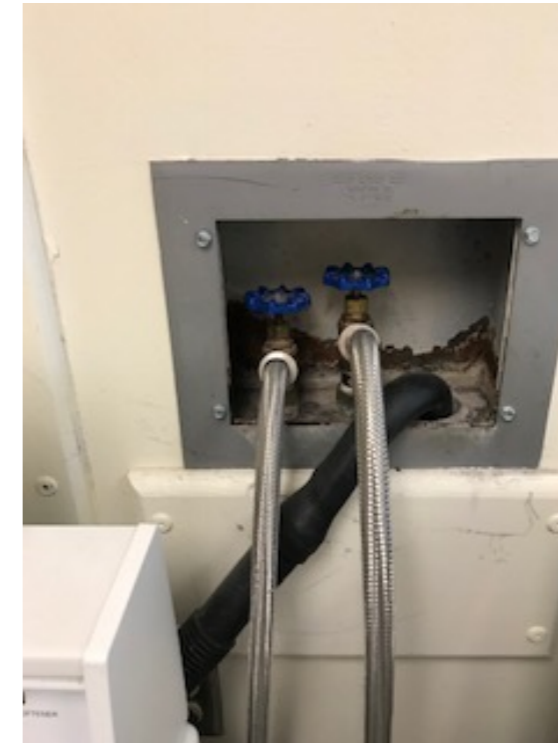
C7-146 (Washer water connections) - Risk H
