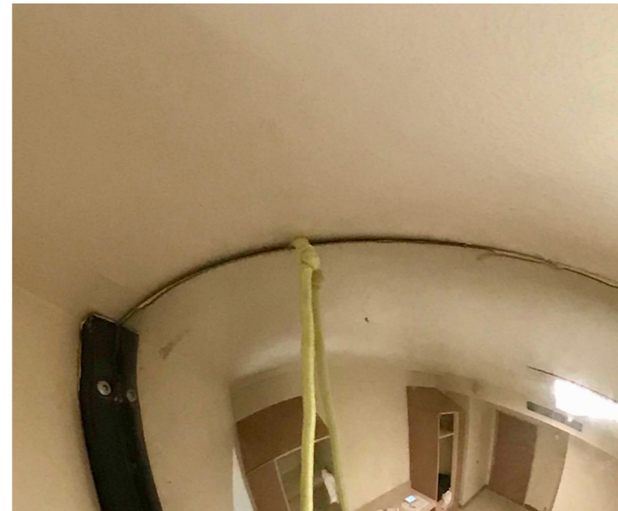
C8-246 (Convex mirrors not flush to ceiling) - Risk H
