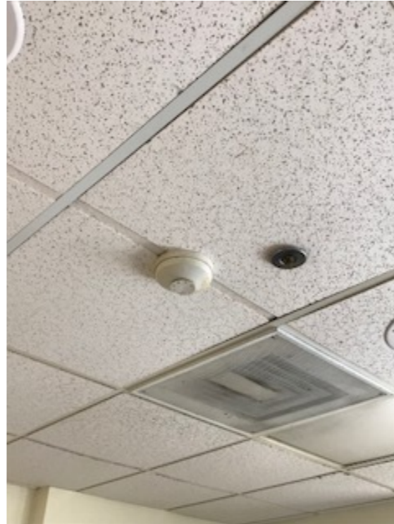
C7-125 (Lay in ceiling & sprinkler) - Risk M
