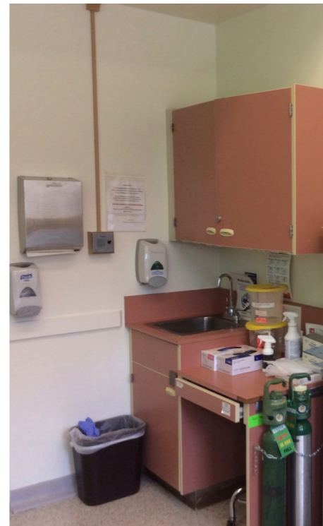
C9-318 (Cabinet hinges, Sink hardware, Paper towel, Hand sanitizer) - Risk H
