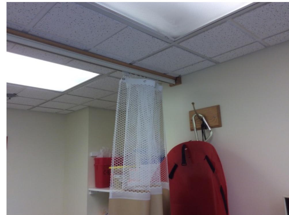
C9-318 (Hook, Curtain glide & Lay in ceiling) - Risk H
