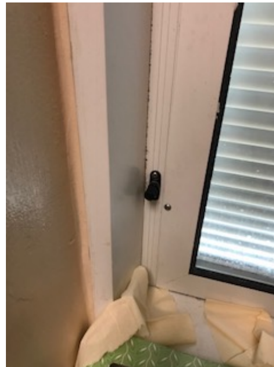
F6-2-26; F2- 2-21 Rooms (Knobs) - Risk H
