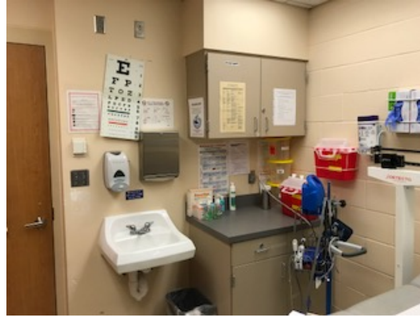
F1- 58 Exam room (Faucet) - Risk H
