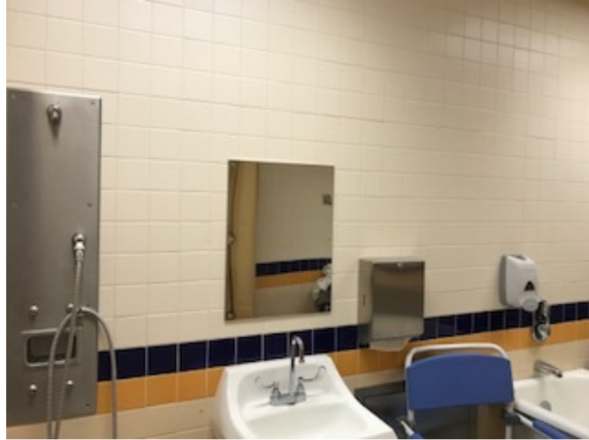
Tub Rooms, all (Faucets fixtures standard, Paper towel dispenser, Mirror not flush, Tub/shower water controls) - Risk H
