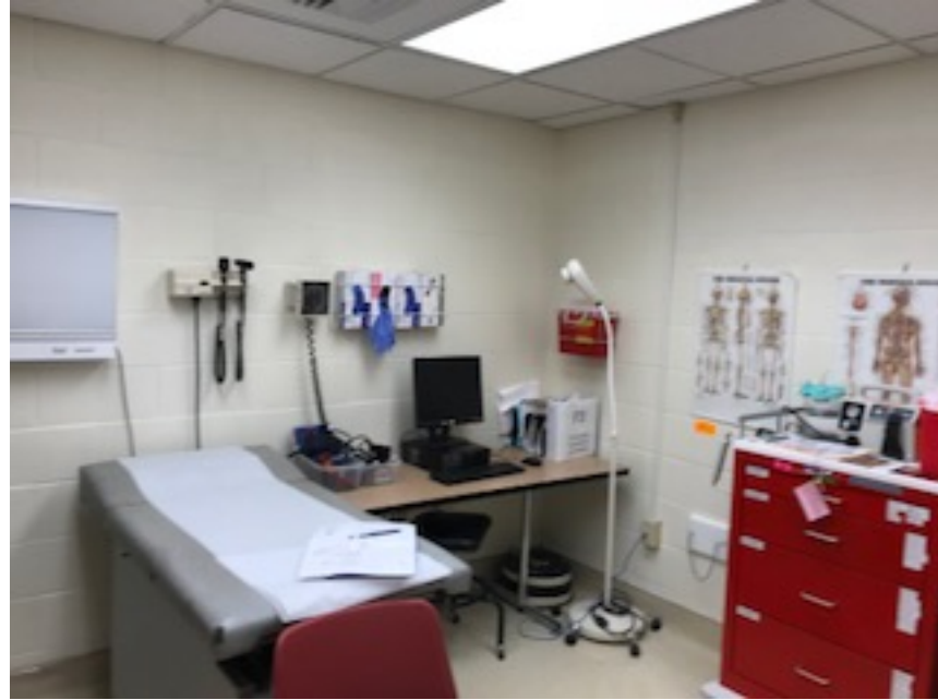
F8; F5; F4 Exam rooms (Medical equipment: otoscope/BP, Viewer, Lamp, Cart, Scale, Portable BP unit, O2 rack and chain, Conduit) - Risk H
