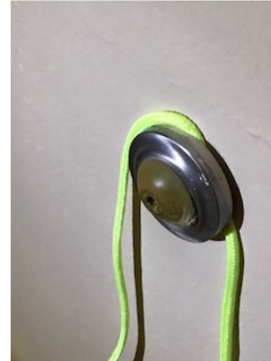
F7- D059; F3- DC59 Interview conference room (Door stop-like kind) - Risk M
