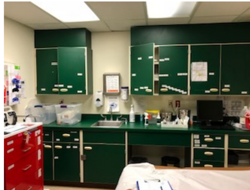
E7-157 (Lay in ceiling) - Risk H
