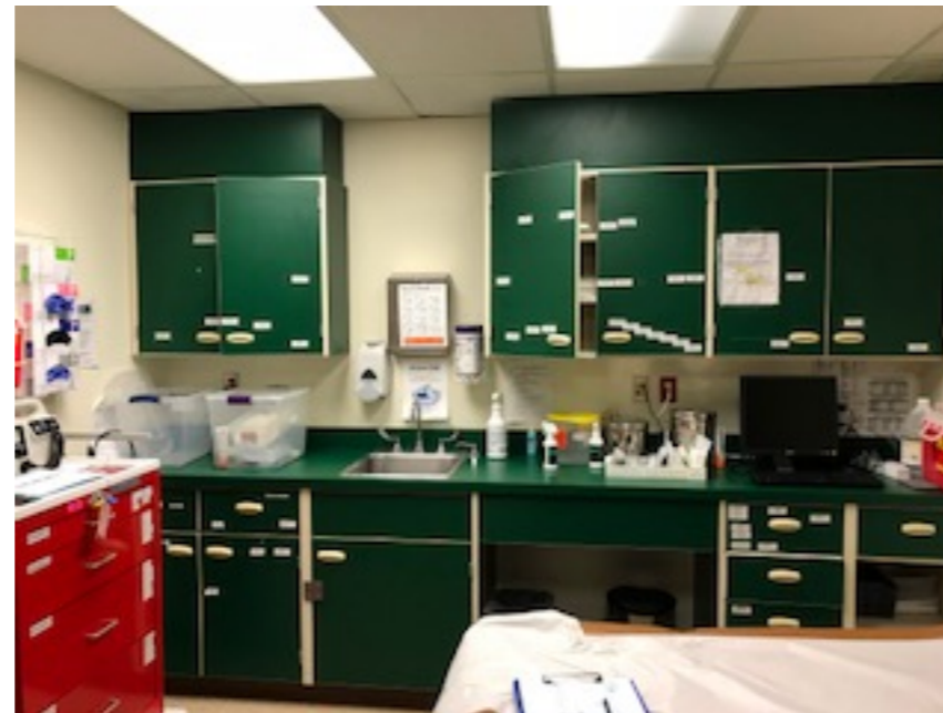
E7-157 (cabinet hinges) - Risk H
