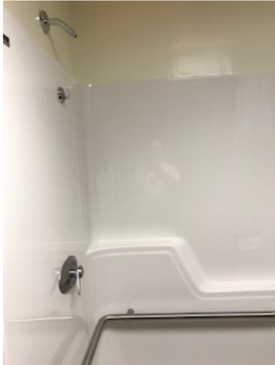
E8-220 (Storage) - Risk H
