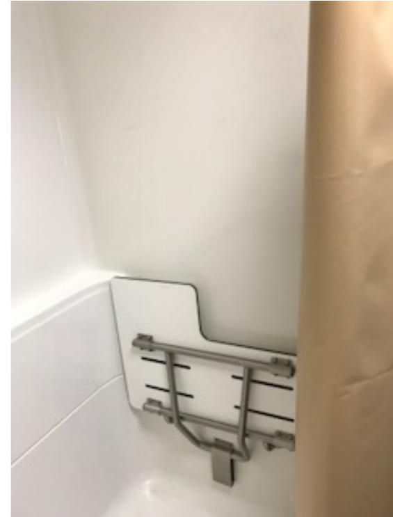
E8-220 (Storage) - Risk H
