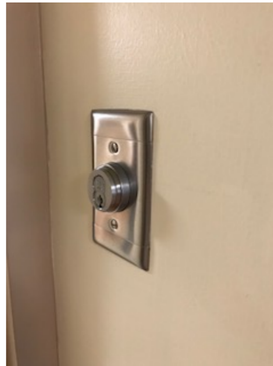
E7- All rooms (Lock) - Risk H
