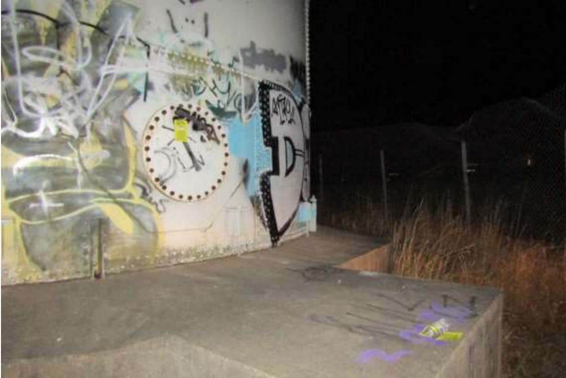
Photo shows the foundation, which is in compliance with AWWA D103-09; 13.5.1: Height above ground and appears to be in good condition.
