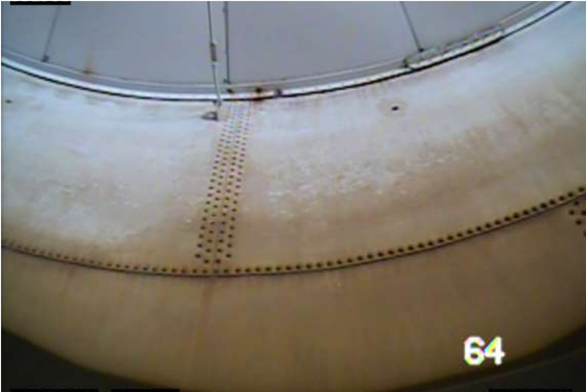
Photo shows the interior roof-to-rim angle connection, which appears to be in good condition.
