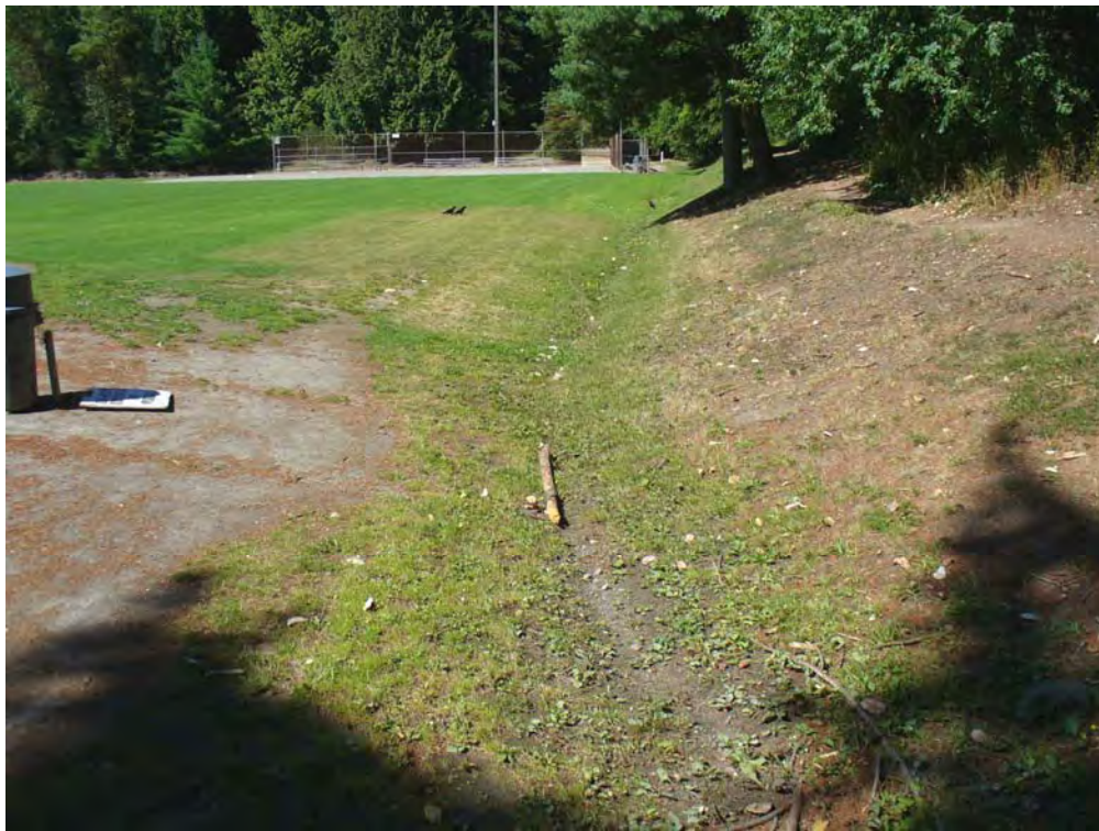
Figure 3. Facing upstream along the east fork of Hamlin Creek in Hamlin Park between the toe of the slope and a baseball field (Taken on 8/4/08).
