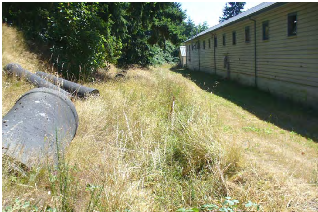
Figure 13. Area B facing downstream. Notice former pipe sections, now removed, and the close proximity of the existing buildings (taken on 8/4/08).
