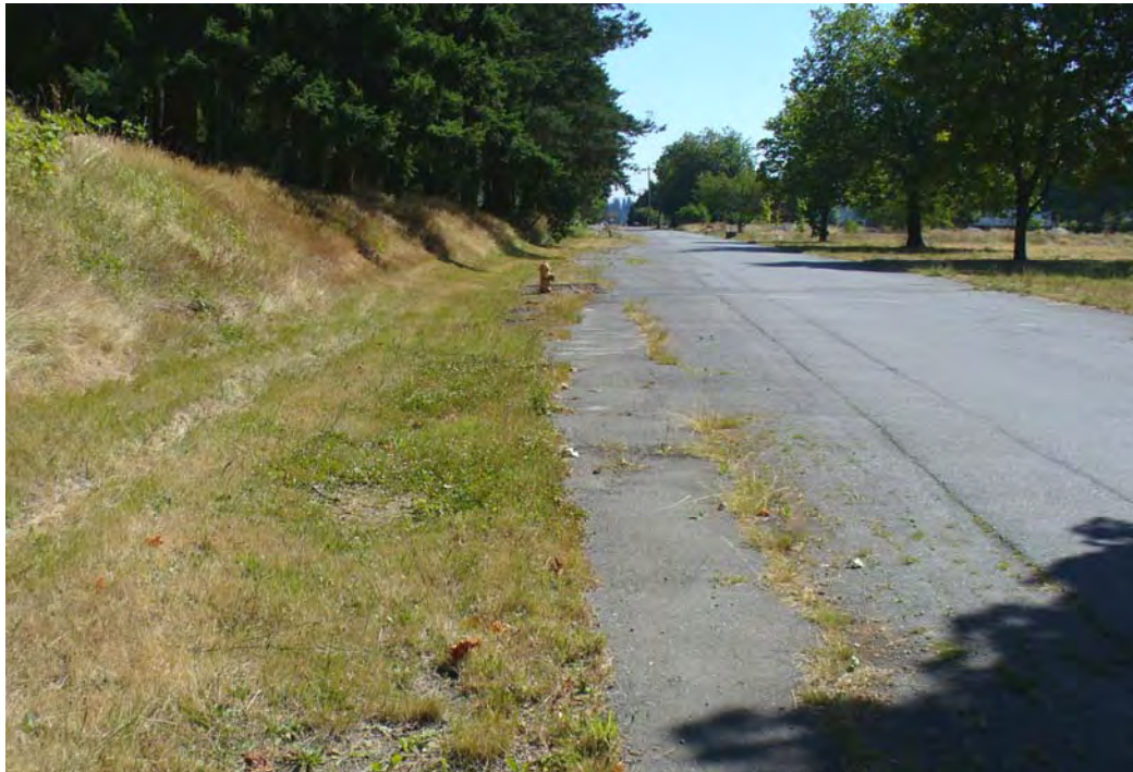
Figure 8. Facing South along the Area A daylighting area, showing toe of forested slope to the left [east] (taken on 8/4/08).
