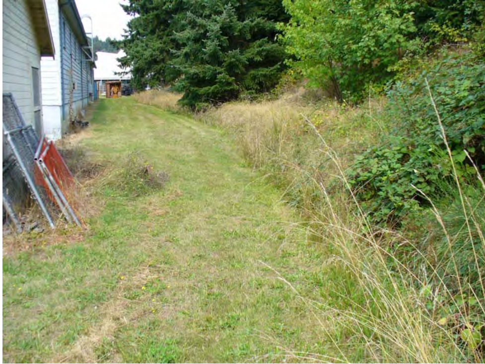
Figure 14. Area B facing upstream. The existing channel is an abrupt, grass-lined ditch. Again, notice the close proximity of the existing buildings (taken on 9/17/08).
