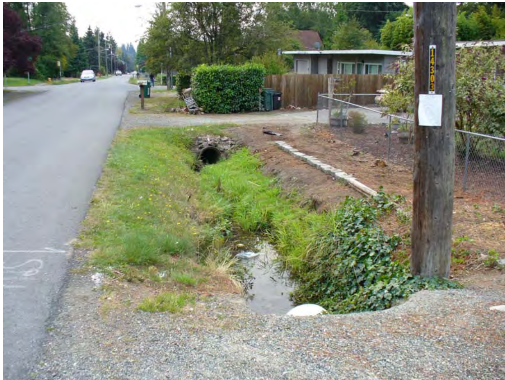
Figure 4. Ditched Hamlin Creek channel along the west side of 20th Avenue NE, downstream of the Fircrest Campus (Taken on 9/17/08).
