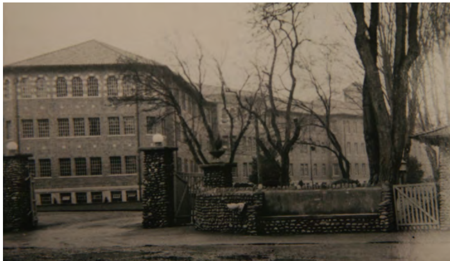
Secondary gate. Photograph courtesy of the Washington State Archives.
