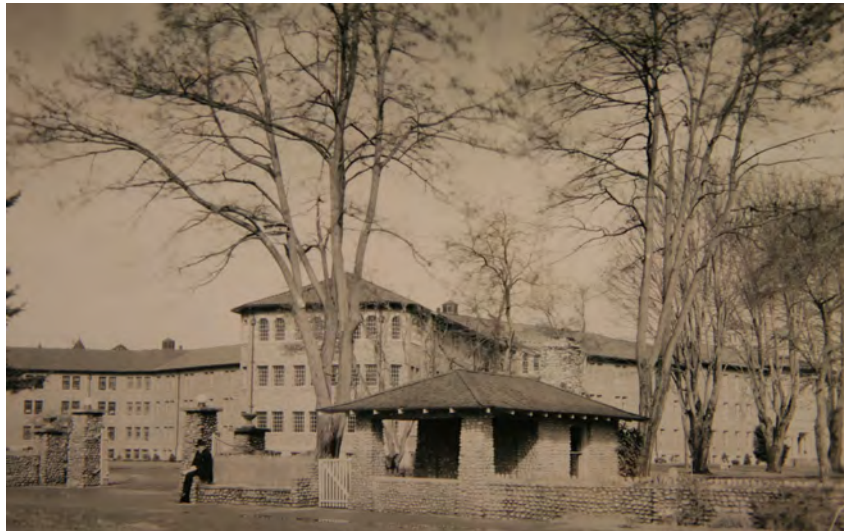
Gate house at main gate. Photograph courtesy of the Washington State Archives.
