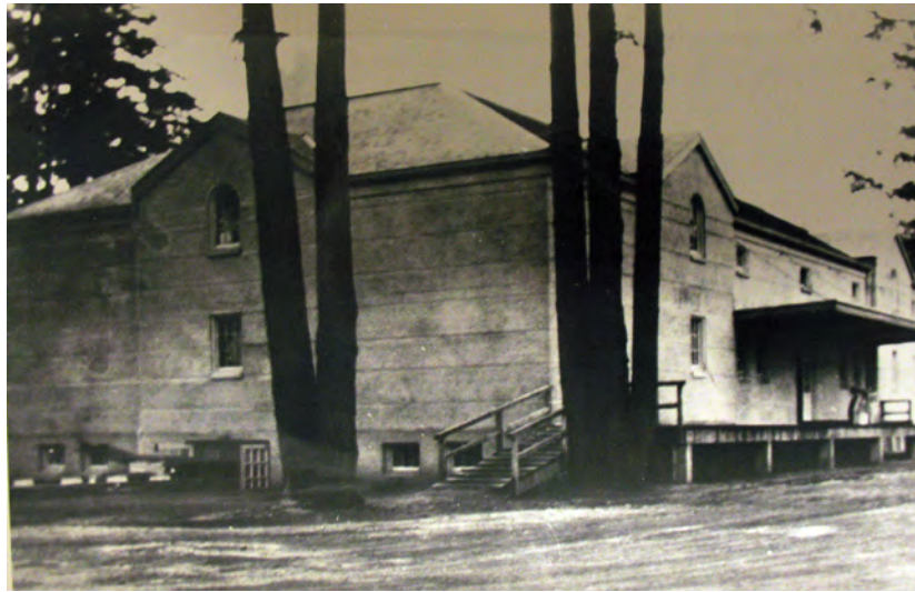
Commissary. Photograph courtesy of Western State Hospital.
