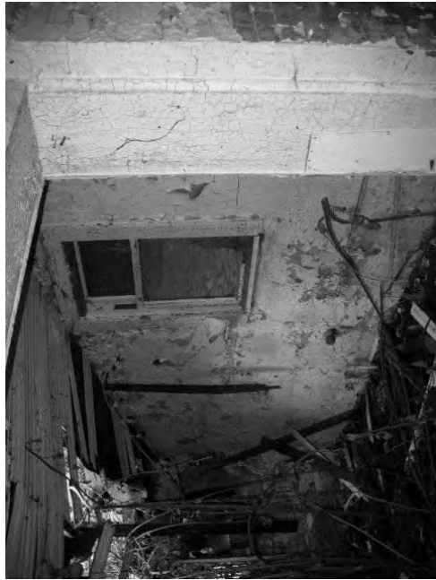
View of interior view of windows.
