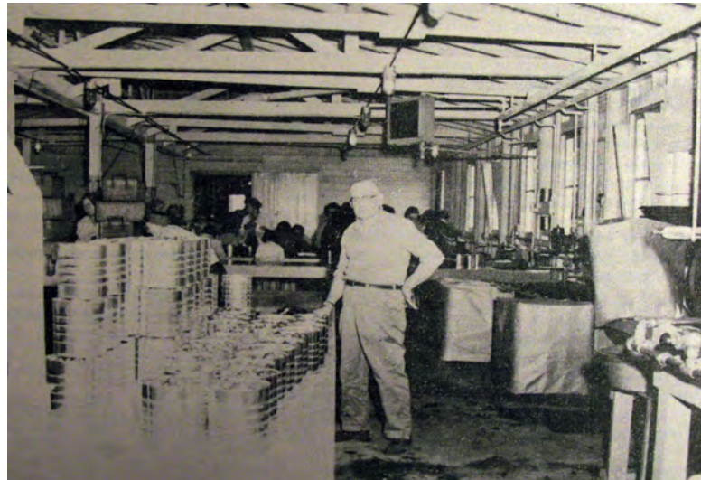
Cannery building interior view. Built as a warehouse in 1937-1938 by 1951 this building had been converted for use as a cannery. Photograph courtesy of the Washington State Archives.
