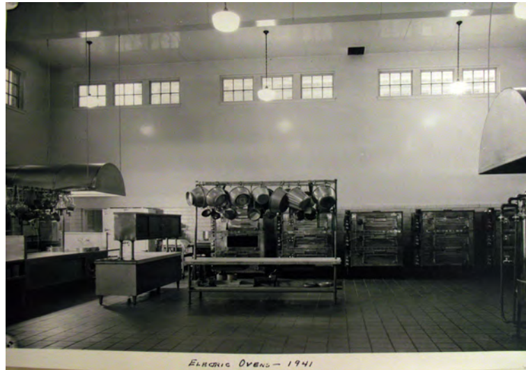
1941 kitchen with electric ovens. Photograph courtesy of the Washington State Archives.
