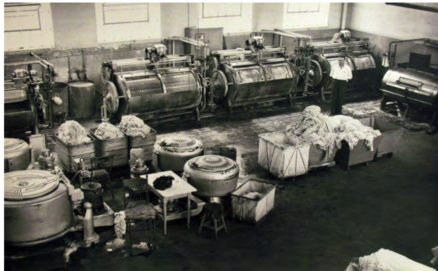
Laundry facilities interior view. Photograph courtesy of the Washington State Archives.
