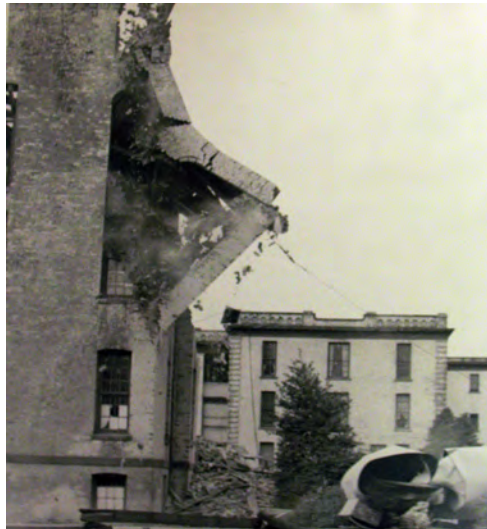
1947 fire damage. Photograph courtesy of the Washington State Archives.
