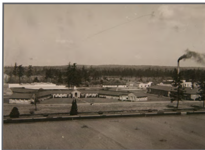
Geriatrics building constructed west of the main hospital grouping. Source: Washington State Archives.
