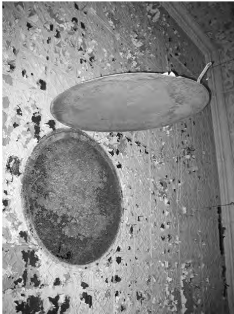
View of door to roof vent.
