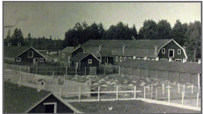
Fencing at the dairy operation. Source: Washington State Archives.
