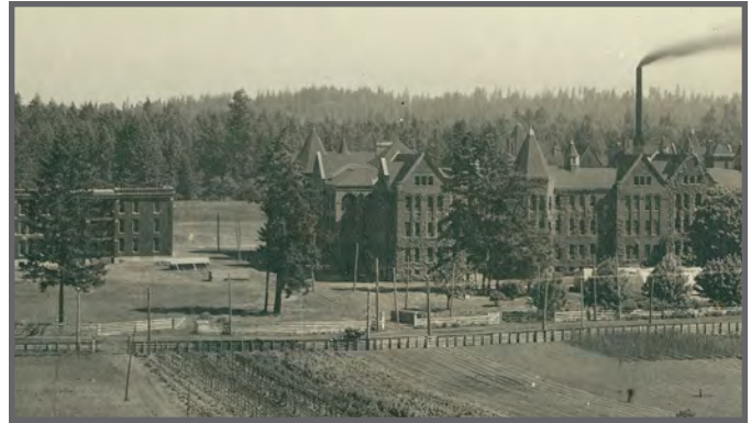
Fencing along Steilacoom Boulevard SW. Source: Washington State Historical Society.
