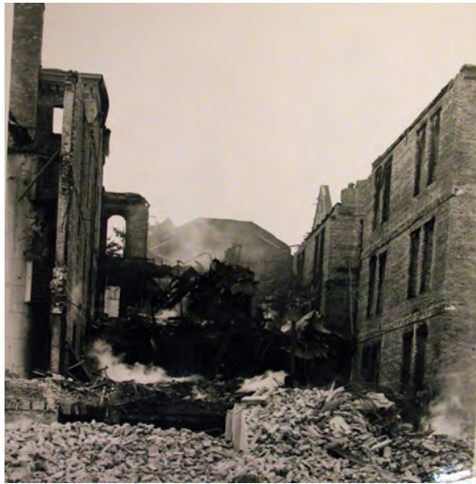
1947 fire damage. Photograph courtesy of the Washington State Archives.
