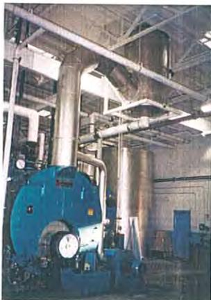
Installation of a DC-2-500 SUPERMIZER servicing a 500 H.P. boiler.
