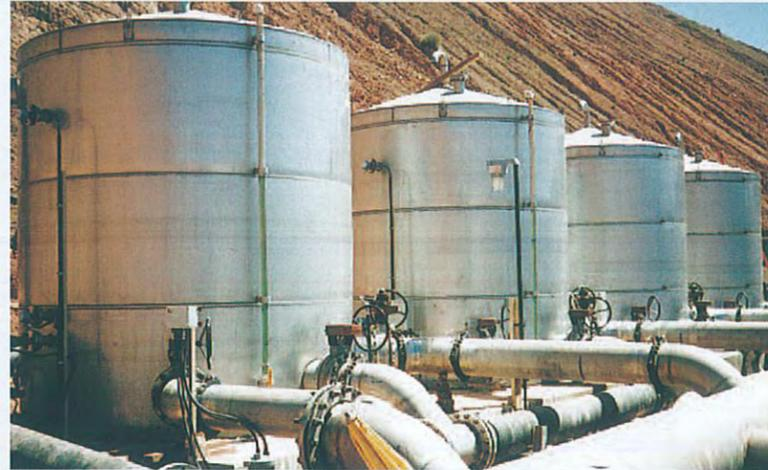
*Four of sixteen 12,000 gallon T-316L stainless steel tanks for acidic leach solution in mining operations for Bechtel Corp.*
