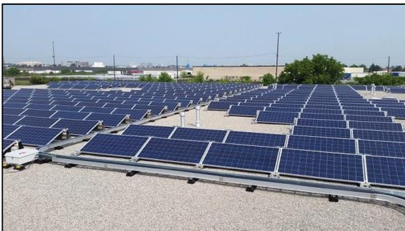
Figure 6: Ballasted racking installation system on flat roof
